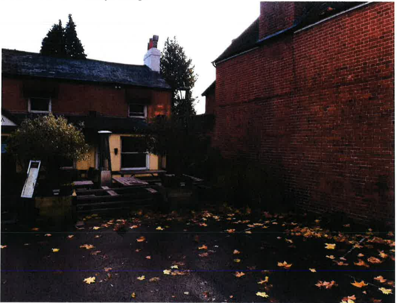
Picture 3 Side of Crossways Cottage
